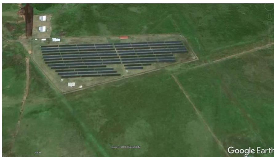
Photo 2-6 The Fighter One Power Station
