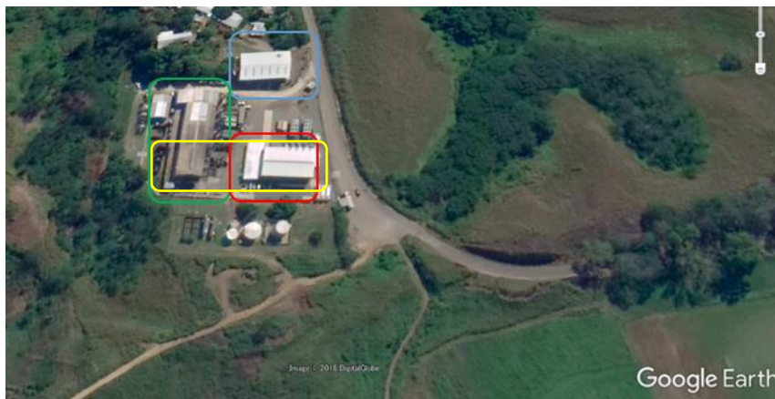
Figure 2-9 The Lungga Power Plant
