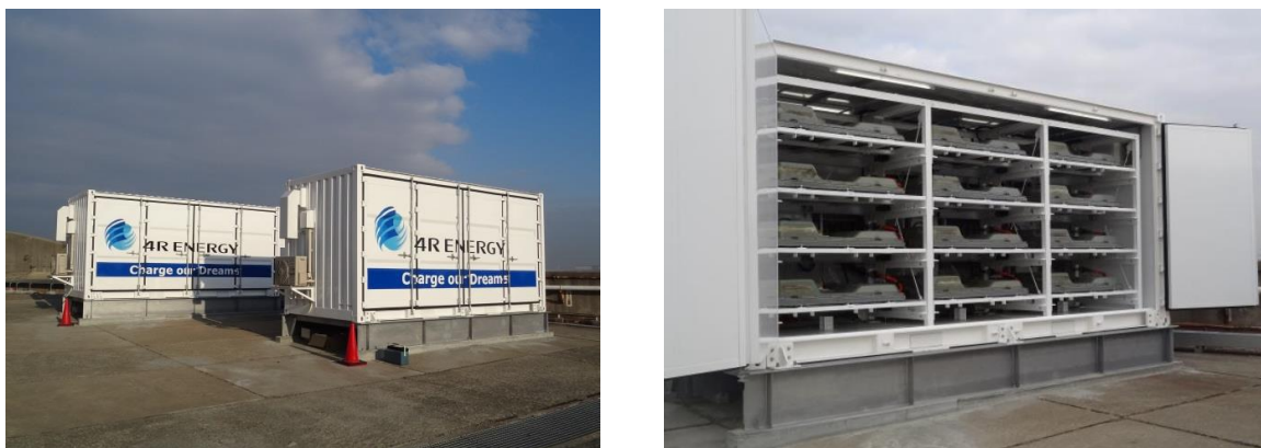
Photo 4-1 Reuse Battery: (left) Exterior, (right) Inside of package
