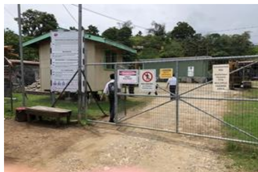
Photo 2-5 The Honiara Power Station
