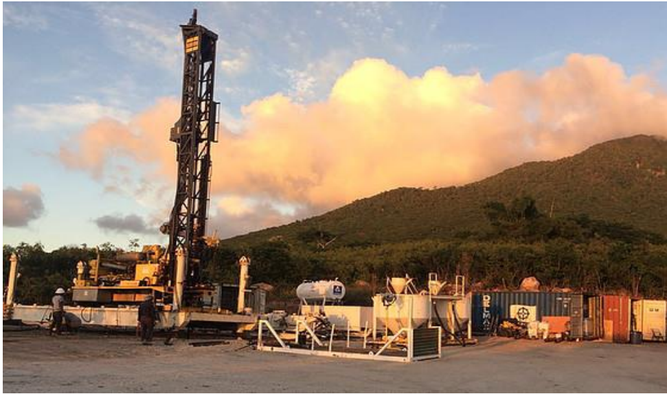
Exploration well (N-4) drilled March 2018, Hamilton Nevis.
