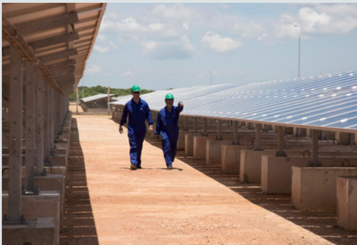
IRENA-ADFD Facility: Grid connected solar PV project, Cuba
